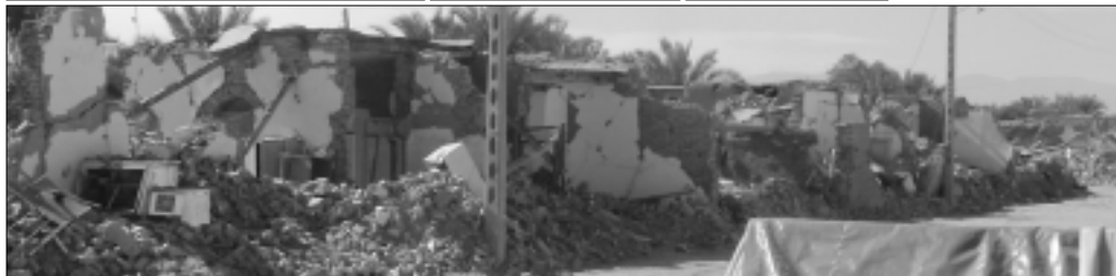
Photos courtesy of FEMA
